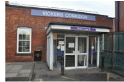
20 Access to Vickers Corridor and wards
